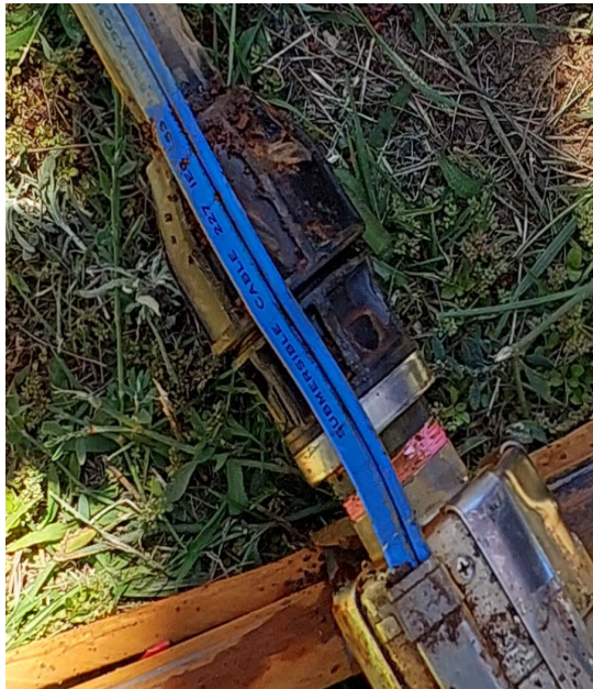
Rural poly fittings as noted on bore cap and pump outlet.
