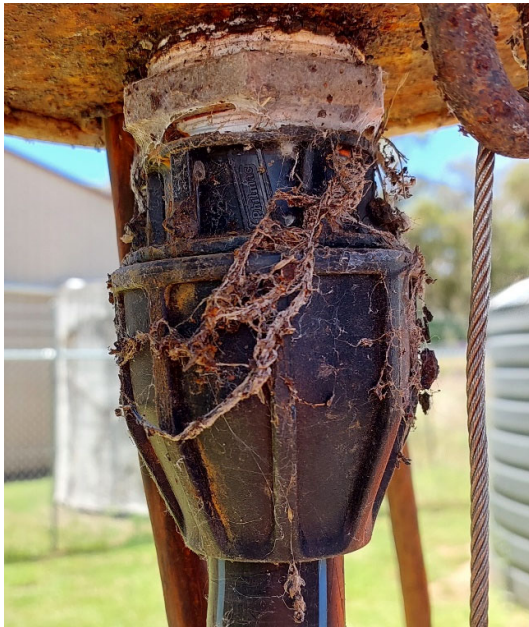
Rural poly fittings as noted on bore cap and pump outlet.
